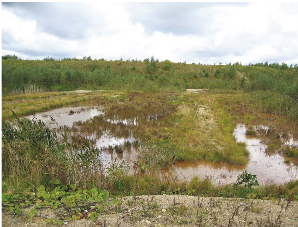
Figure 14. An environmental permit decision can contain provisions on measures to be undertaken after discontinuing operations, such as covering and landscaping a tailings area or treatment of discharge from storage areas. The tailings area at Keretti mine in Outokumpu has been covered and revegetated (background). There is an aerobic wetland for treatment of the discharge from the tailings area (foreground).
