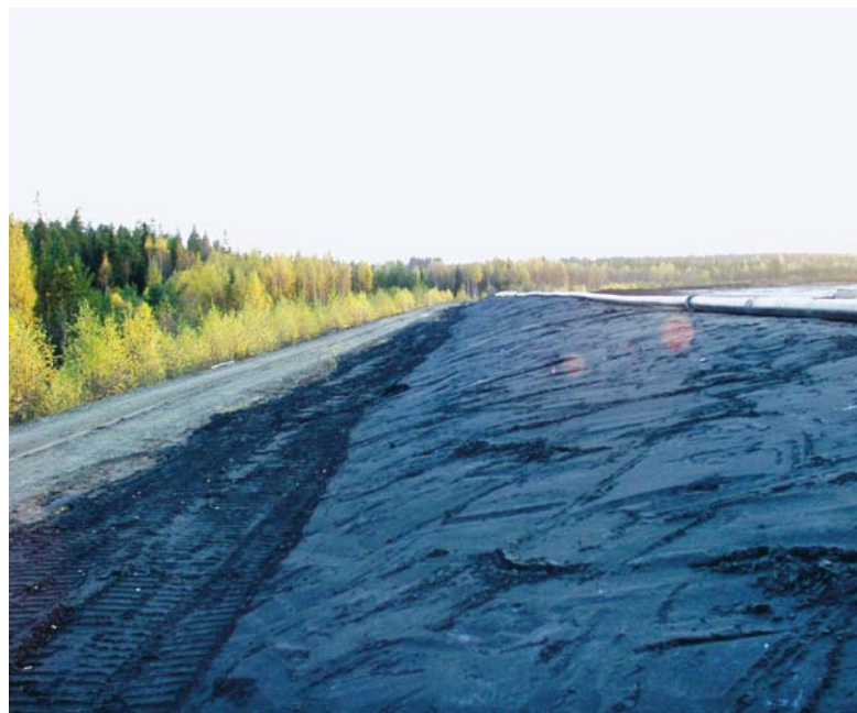
Figure 38. Tailings can be used for various purposes during mining, such as increasing the height of retaining embankments surrounding tailings impoundments.
