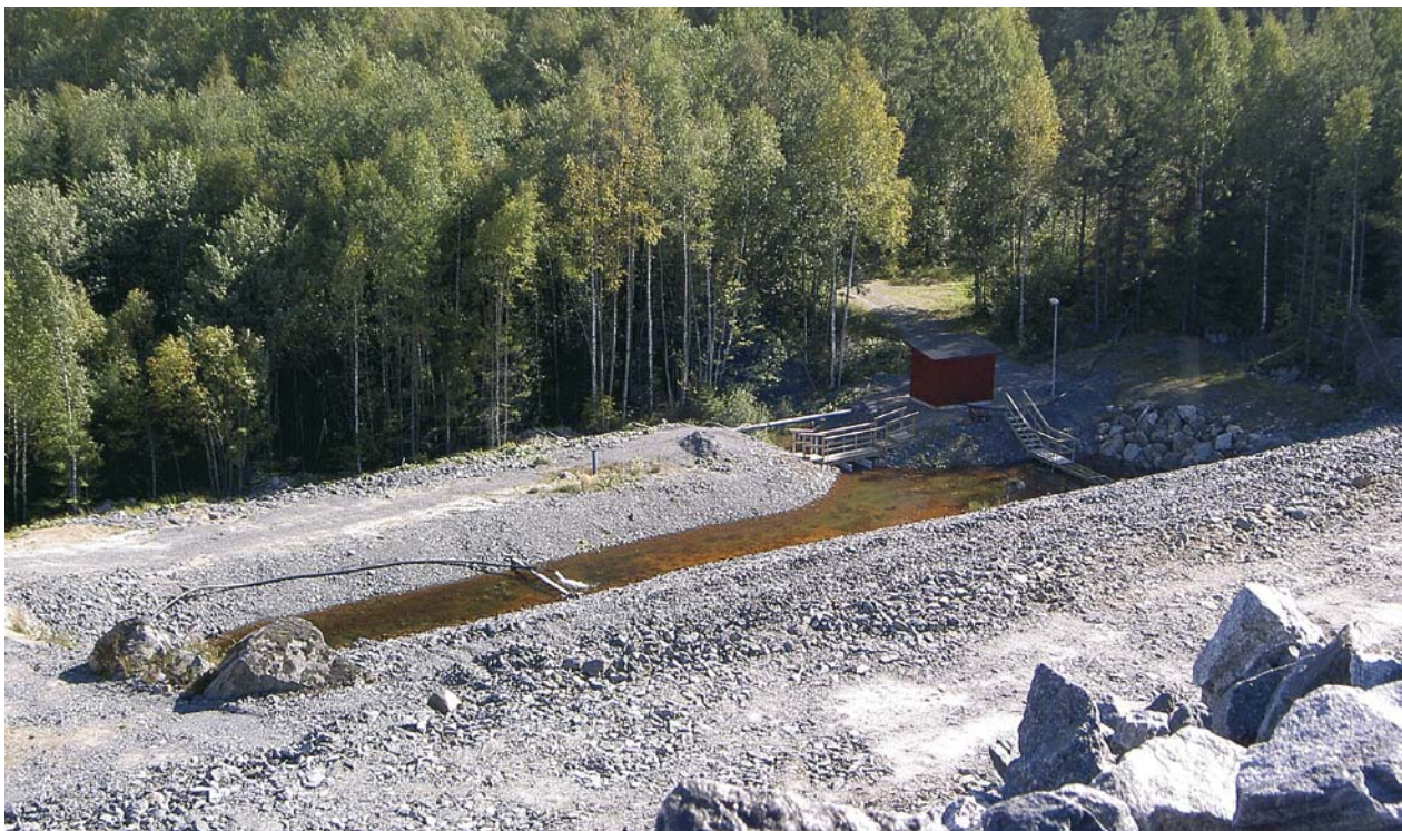
Figure 44. Potential seepage of water through tailings dams is contained by an effective system of trenches, which also channels water for further treatment as necessary (Zinkgruvan Zn-Pb mine, Sweden).
