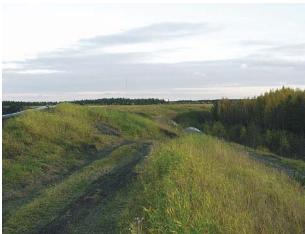
Figure 12. It is possible to commence landscaping and covering of tailings concurrently with mining activities, which facilitates integration of the mine area with the surrounding environment. Covering in this way also serves to inhibit oxidation of sulphide-rich tailings (Landsaped tailings embankment, Hitura nickel mine, Nivala, Finland).
